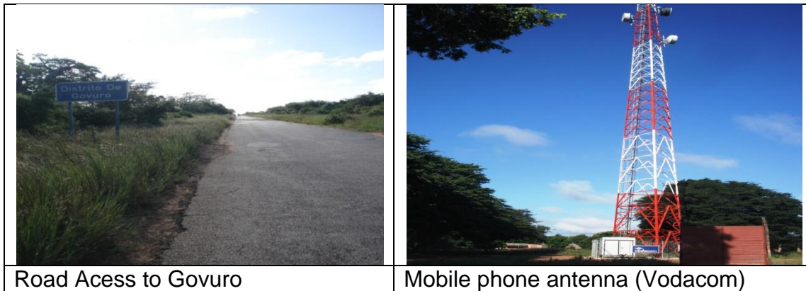
Figure 5. Transport and communication infrastructures
